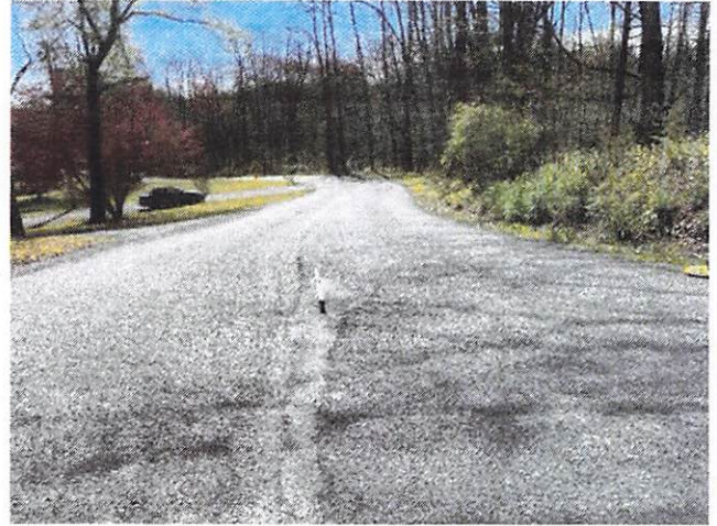
Exhibit 6 – Eastbound approach to the Site Driveway
